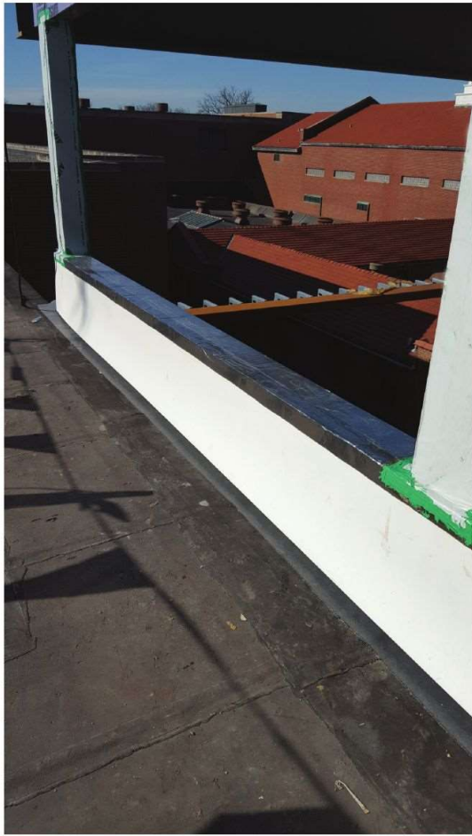
Proper installation of transition membranes at the roof and window opening.
