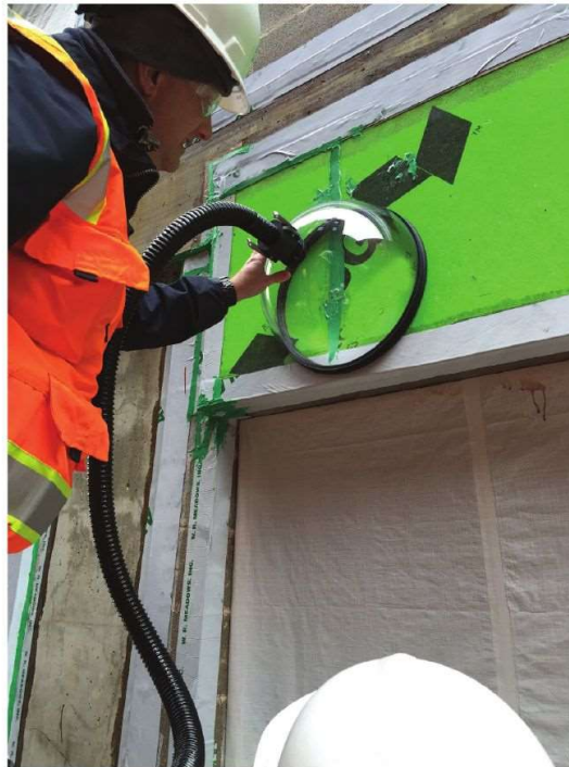
Performing ASTM E1186 on a fastener and detail strip edge.
